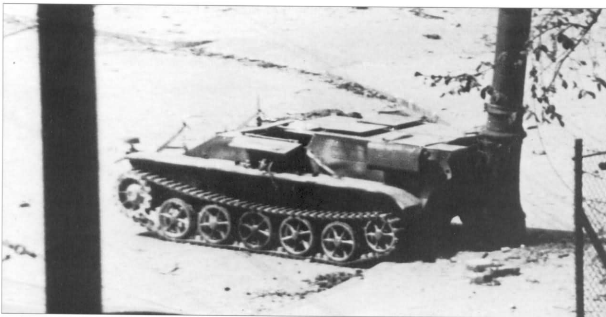
A Borgward B IV Ausf.C (Sd.Kfz.301) demolition vehicle from Pz.Abt. (FKL) 302 sits abandoned on a Warsaw street in August/September 1944, where they were used extensively against Polish partisans hidden in buildings and behind barricades. The Borgwards were radio controlled from a command vehicle, in this case a StuG.III Ausf.G, which guided them to their target where a 500kg explosive charge was dropped. The Borgward was then backed away a safe distance and the charge detonated. On this one, the charge is missing. A camouflage paint scheme can be made out along with the load class shipping stencil on the side.
