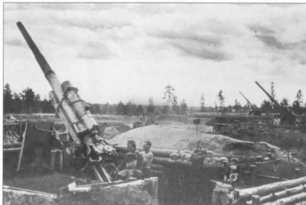
A battery of 8.8cm FlaK18 anti-aircraft guns set up in well emplaced positions in August 1944. As the front approached closer to Germany's borders, anti-aircraft units such as this were forced to evacuate these well prepared positions and become part of a mobile defense against both air and ground targets. These ones are painted dark sand and have white battery markings on the recuperator housing.
