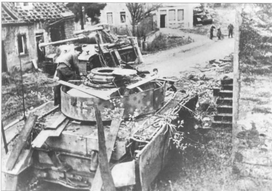
Two photographs of a Pz.Bef.Wg.V Panther Ausf.G from an Army Panzer-Division. It has several rows of spare track links hanging from the side of the turret to bolster its armor protection which was common during the later stages of the war. The white outline tactical number 'IIA1' indicate it is a staff vehicle in second battalion.
