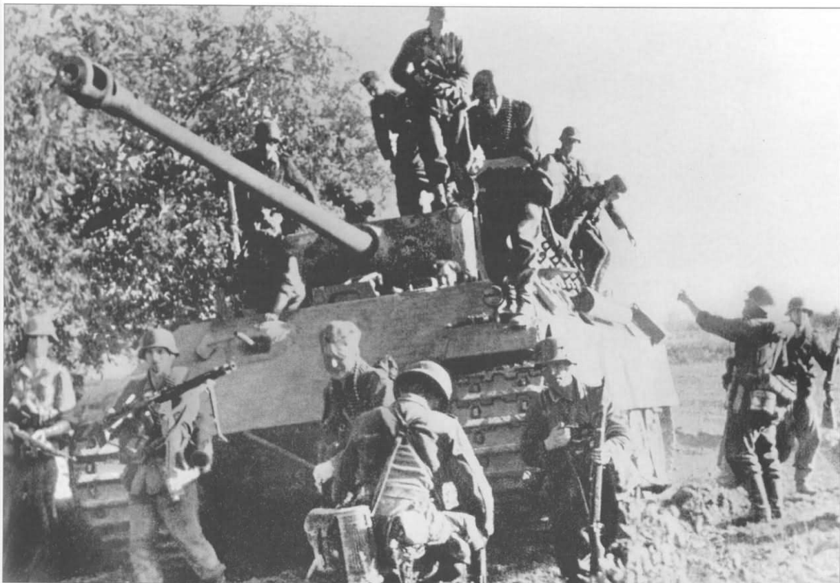
An infantry machine gun squad dismounts from a Pz.Kpfw.V Panther Ausf.G somewhere in Poland during the late summer of 1944. The Panther appears to be fairly new and has zimmerit coating. In early September, zimmerit was dropped along with the requirement to paint the vehicles with dark sand paint. The assembly plants were ordered to apply light patches of camouflage paint directly over the vehicle leaving much of the red oxide primer exposed.
