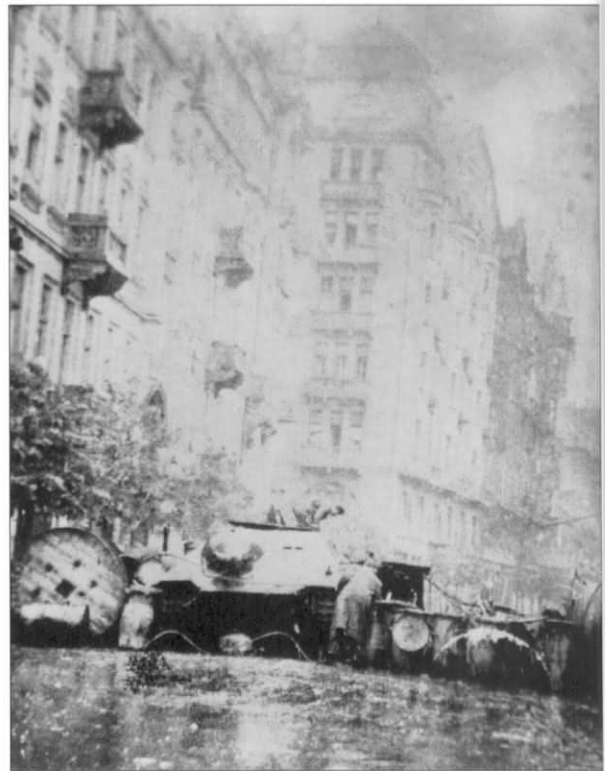
A pair of Jagdpanzer 38(t) 'Hetzer' tank destroyers used by the Germans against the Polish underground army in Warsaw at the beginning of August 1944. Production of these vehicles started in April 1944 and by July 1944, the first combat units began to receive them. They are painted in dark sand with a two color camouflage scheme of green patches with a dark brown outline, best seen on the lead vehicle in the background.
