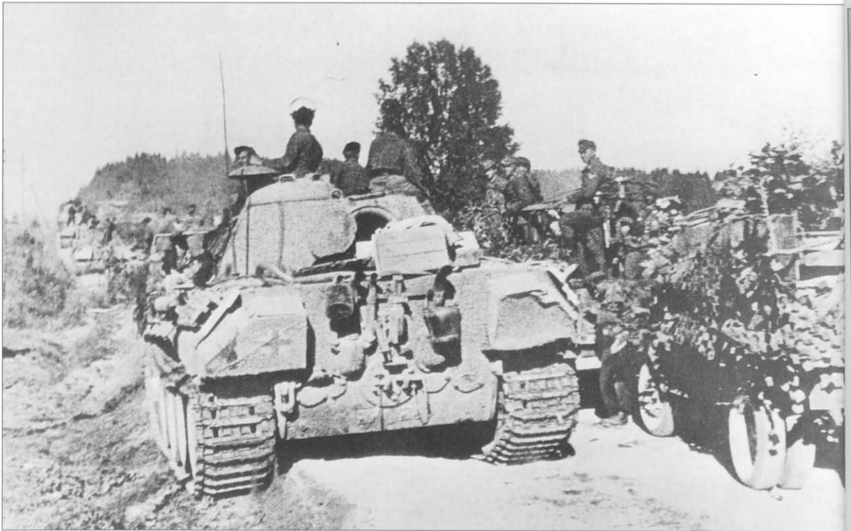
A column of Pz.Kpfw.V Panther and transport vehicles of all types on the retreat somewhere on the Eastern Front, summer 1944. The closest one is a Ausf.A and is fitted with the twin cooling pipes on the left side exhaust that were introduced in January 1944. Mud thrown up on the rear of the stowage bin has almost obscured the Balkenkreuz painted there.
