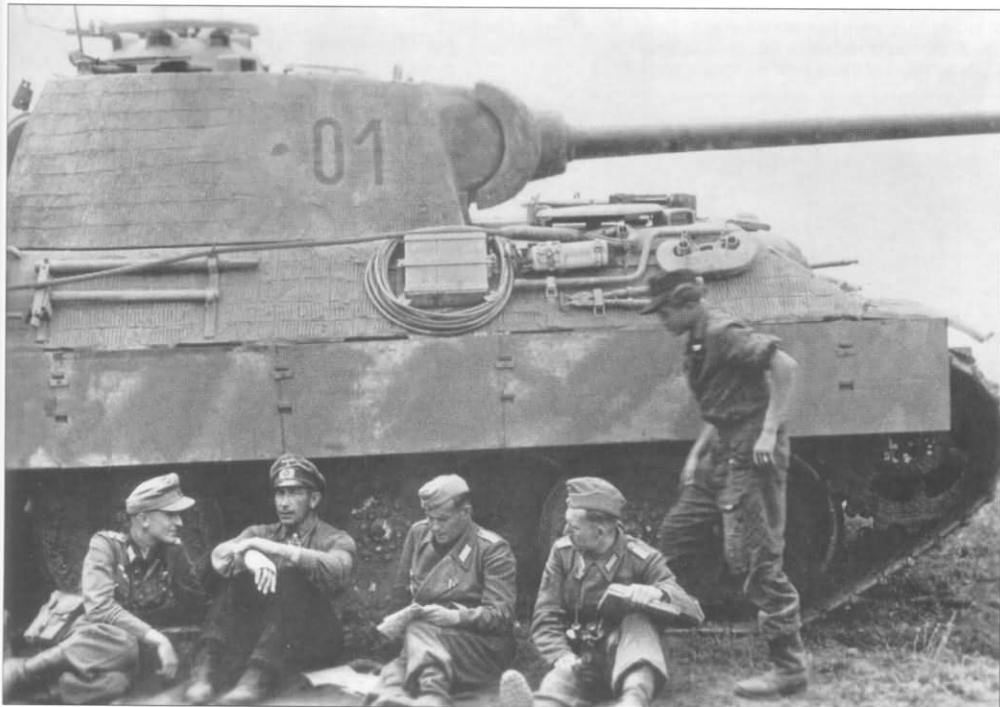
An infantry machine gun squad dismounts from a Pz.Kpfw.V Panther Ausf.G somewhere in Poland during the late summer of 1944. The Panther appears to be fairly new and has zimmerit coating. In early September, zimmerit was dropped along with the requirement to paint the vehicles with dark sand paint. The assembly plants were ordered to apply light patches of camouflage paint directly over the vehicle leaving much of the red oxide primer exposed.
